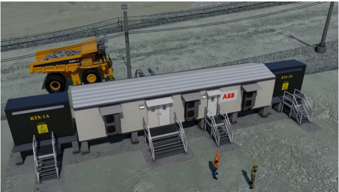
Figure 13: ABB trolley assist system for Copper Mountain in Canada
